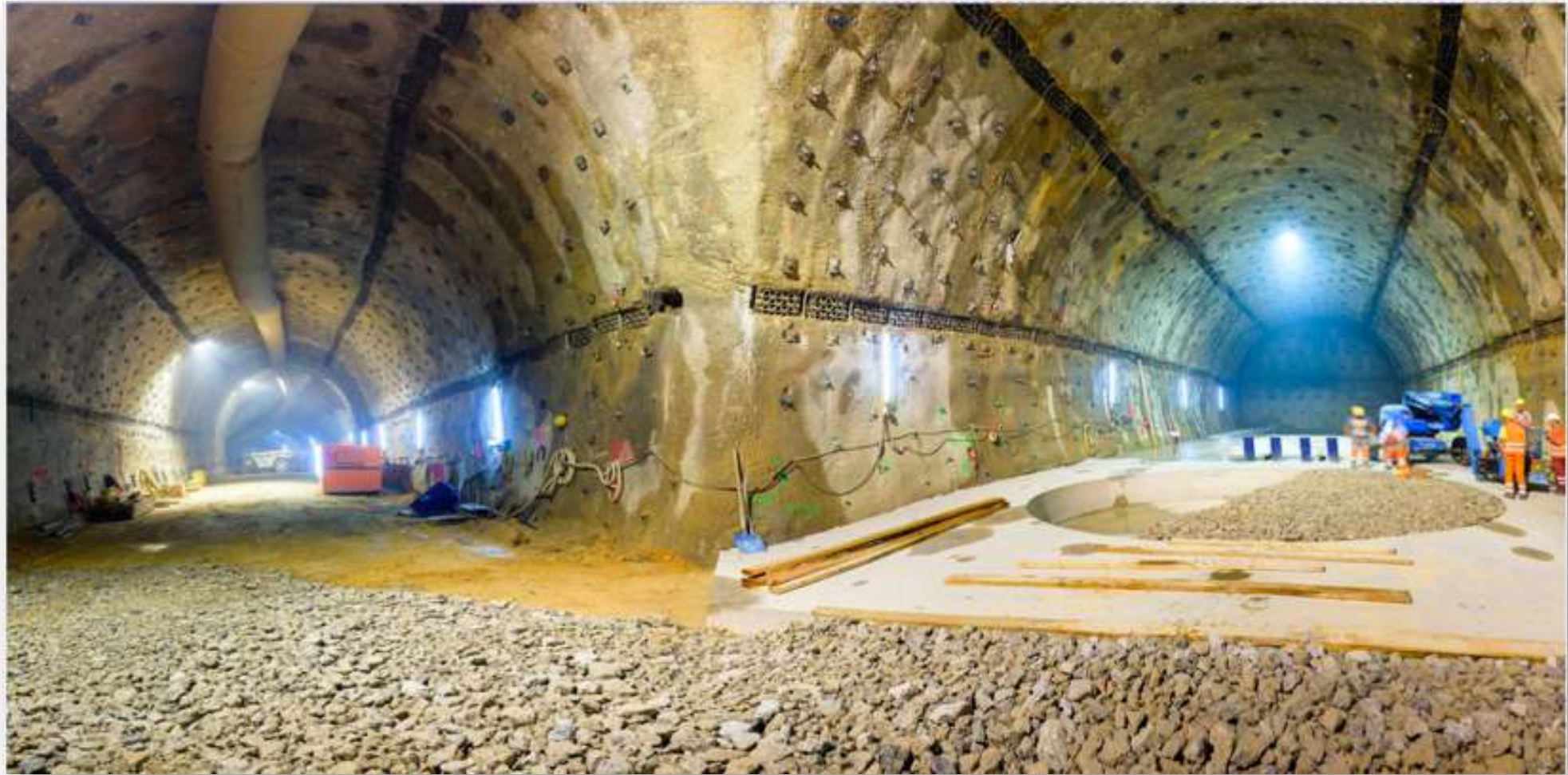
Ongoing excavation and consolidation activities on the 27.2 km long railway tunnel.
