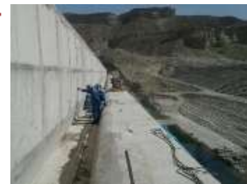
Gravity dam, Iran
