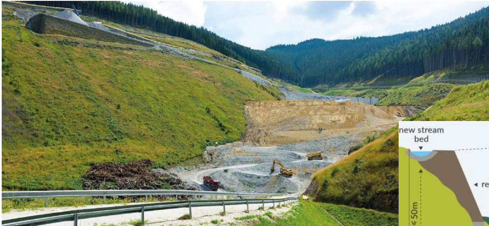
Longsgraben disposal site during the Semmering Base Tunnel excavation
