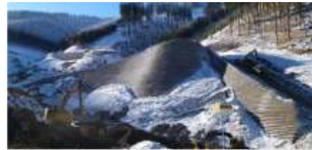
Tunnel construction, AT
