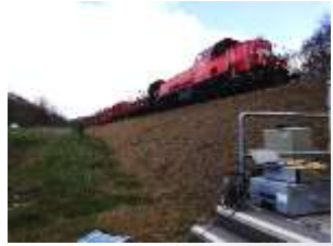
Railway embankment, DE
