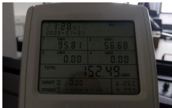
Figure 3.6: Actual power reading on a power meter
