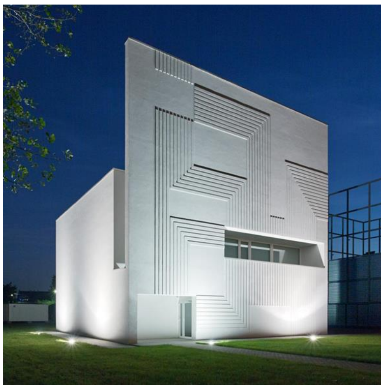
Figure 3.3: External View of the NIFF Data Centre [DATACENTRE]
